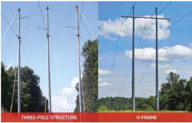
Figure 2-5: Representative typical structures
